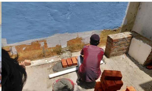
Student carrying out brick masonry work during Skill Lab–III, focusing on mortar application and proper alignment of wall units.
